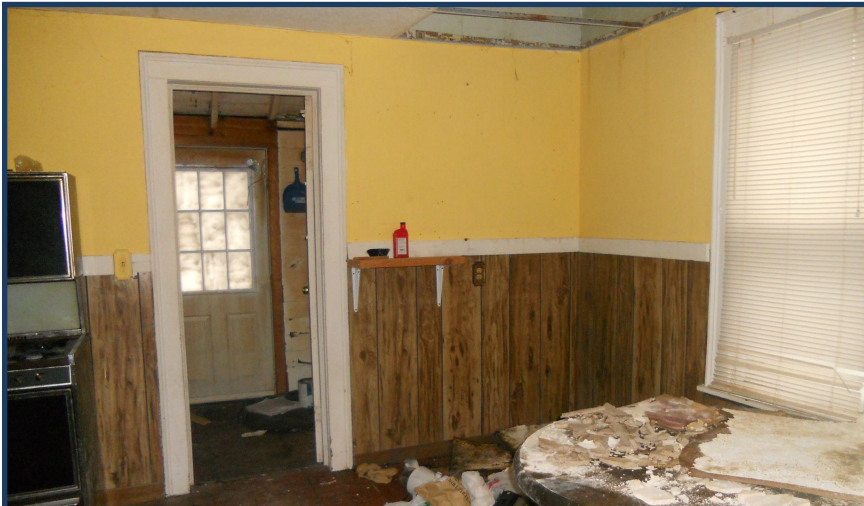
BEFORE: Interior of 1811 Butternut Street prior to renovation
