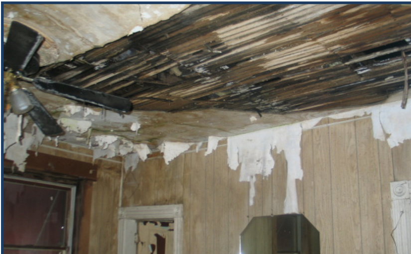
BEFORE: 13 Chambers Street Interior prior to renovation
