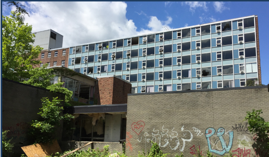
BEFORE: 50 Front Street, prior to demolition
