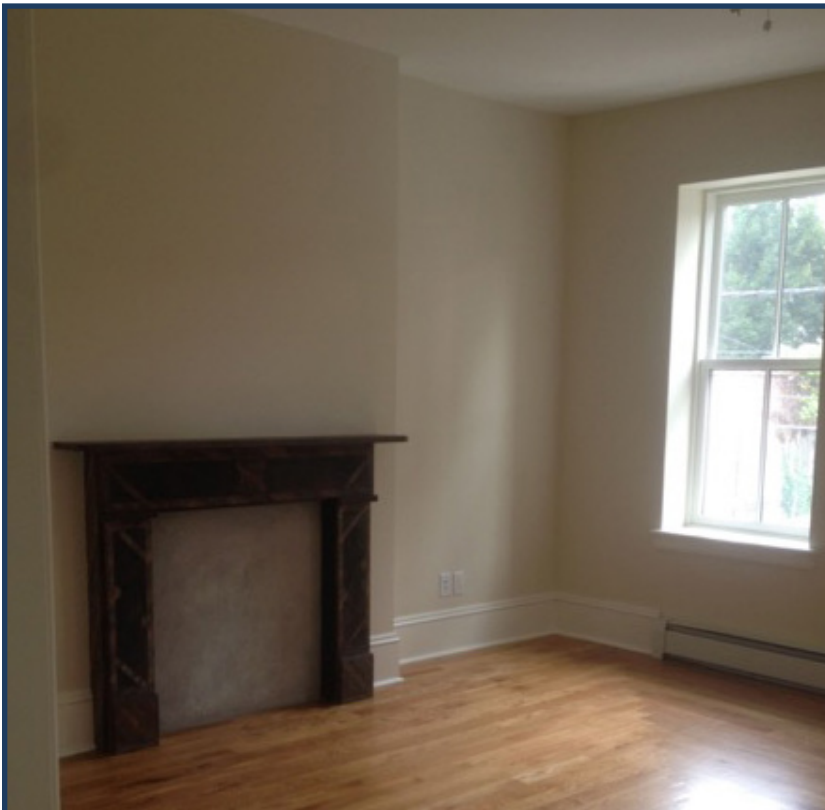
AFTER: Renovated interior of 13 Chamber Street
