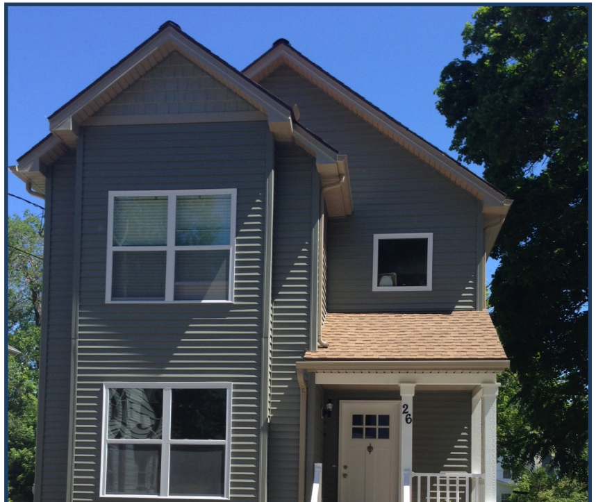
AFTER: New home at 26 Strohm Street, Rochester, NY
