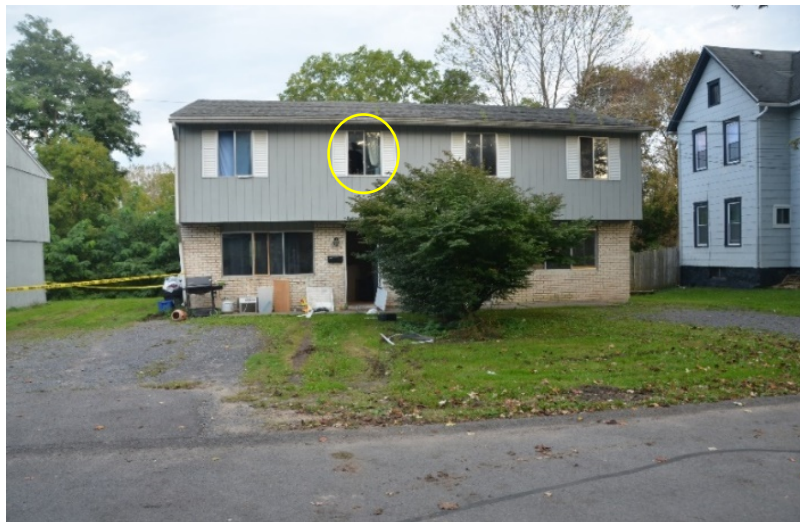
12 Wheeler St. is the left-side apartment in this house. The window Ms. Baida was firing from is circled in yellow. The right-side apartment (10 Wheeler St.) was vacant at the time of the incident.
