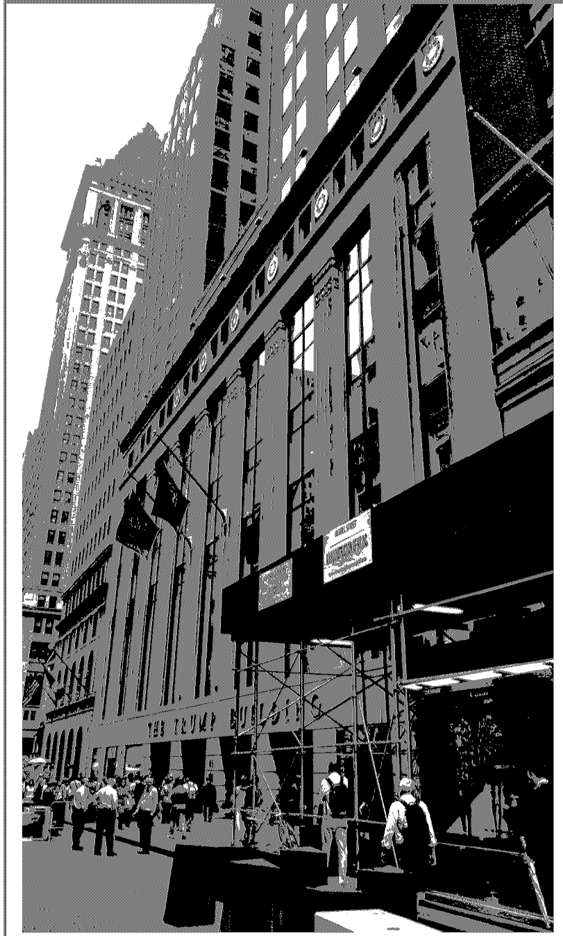
VIEW OF 40 WALL STREET FROM STREET
