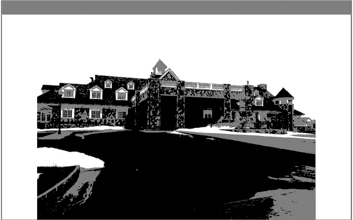
Front view of clubhouse
