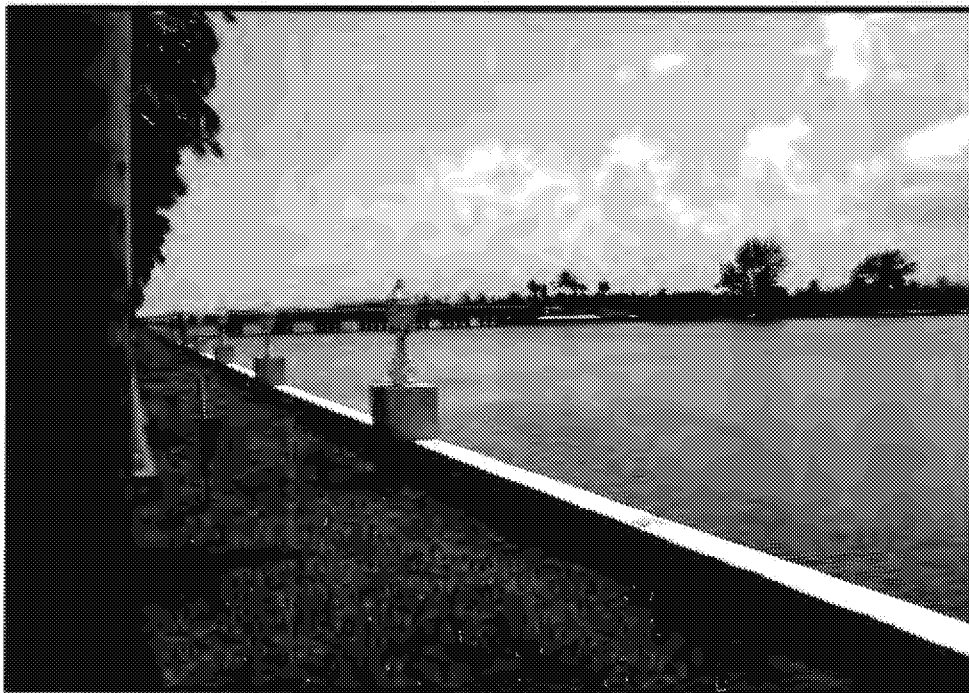
SEAWALL ON OCEAN.
