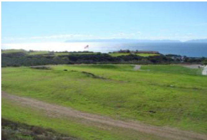
Southeast over partially graded Tract 50667 lots from Palos Verdes Drive South
