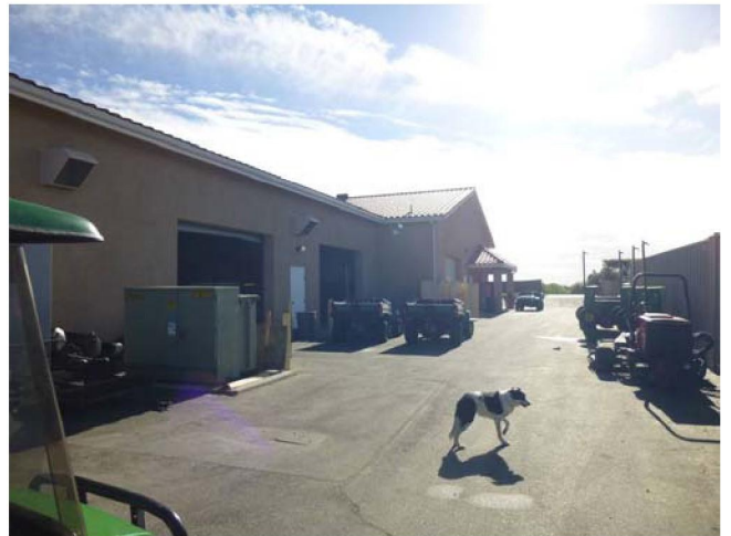
View of Maintenance Facility
