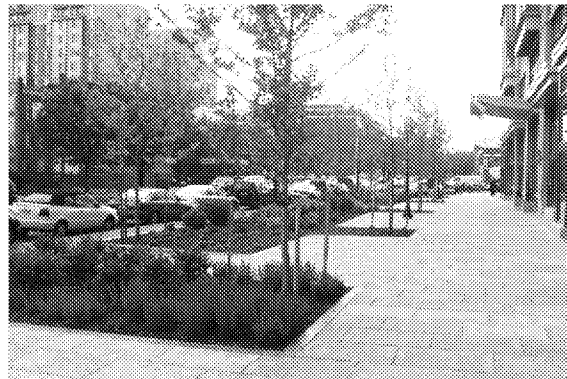
K Street Renovation Washington, D.C.
