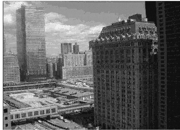
90 West Street Building, New York, NY
