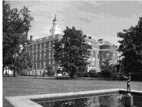
Restored Exterior - Rear Façade, Baltimore, MD
