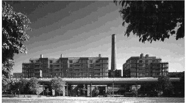
Georgetown Incinerator, Washington, D.C.
