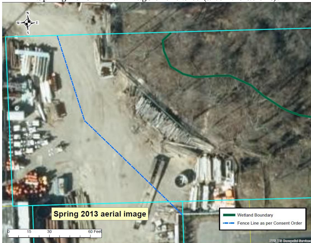
Spring 2013 Aerial Image of the Site (after violations):
