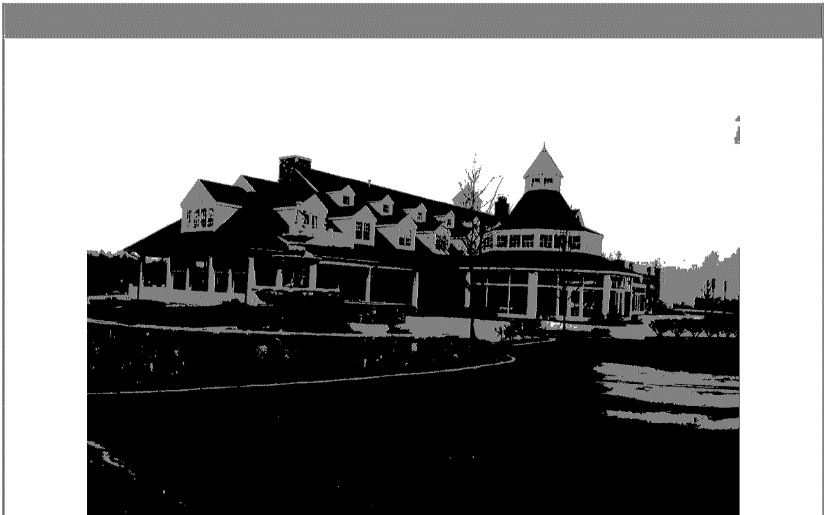
Rear view of clubhouse
