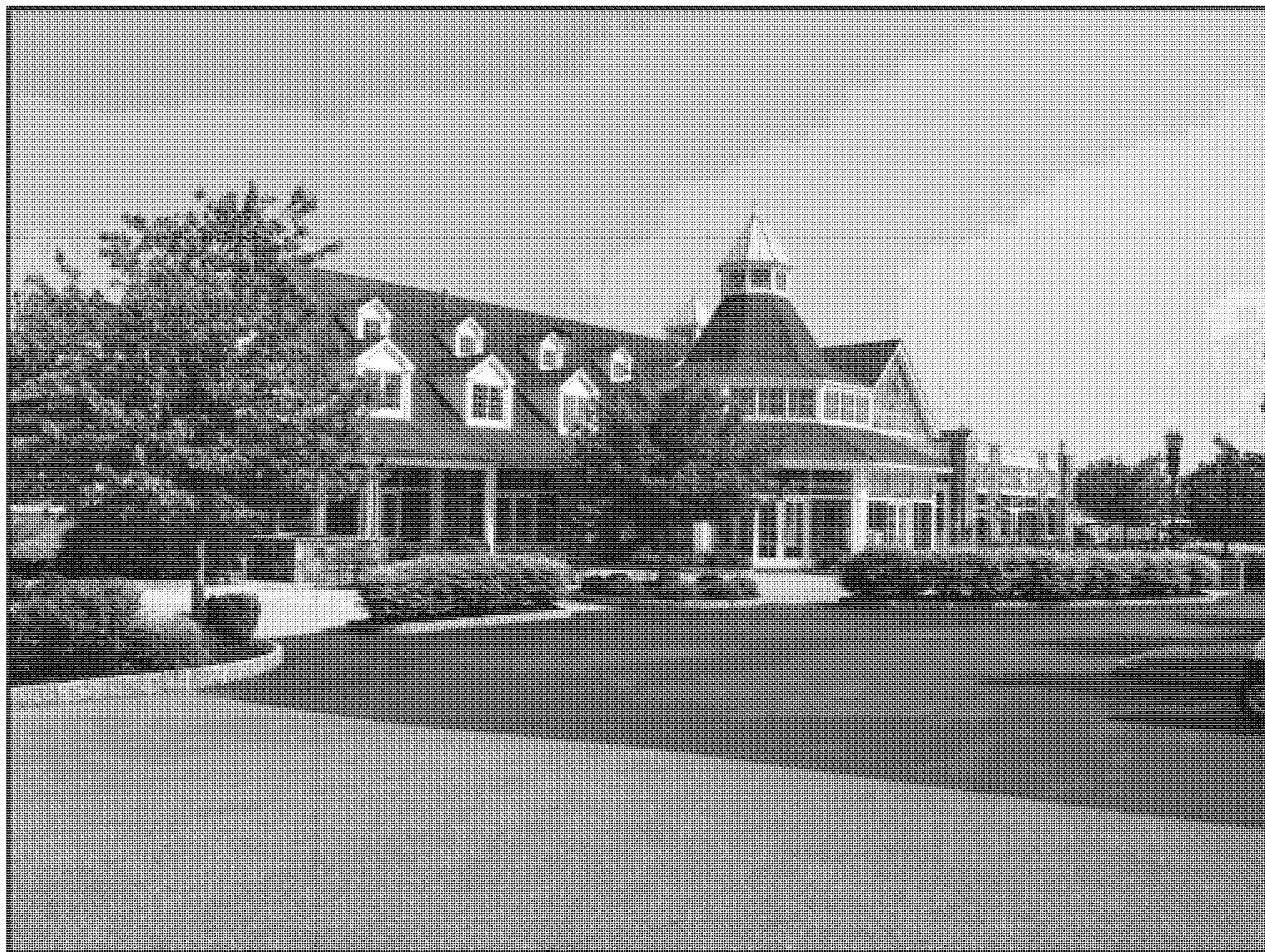
Rear View of Clubhouse
