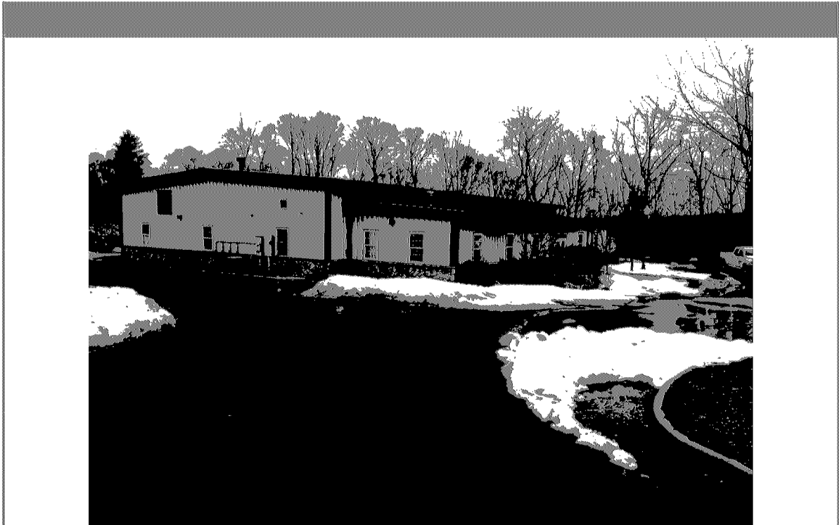
View of maintenance building
