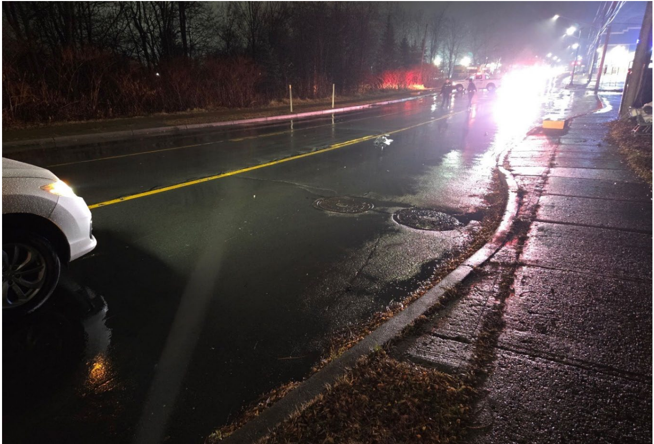
Photographs taken by Cpl. Stackhouse of the roadway
